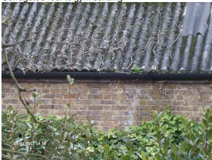
Corrugated roof to gym building
