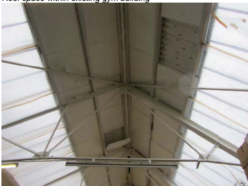
Roof space within existing gym building
